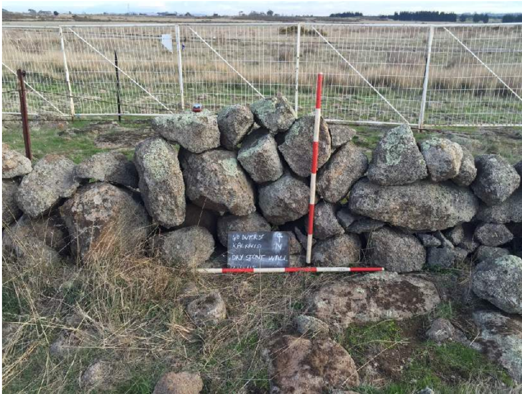
Midsection of Wall No 2 at 40 Dwyer Street Kalkallo which is partly collapsed looking south (27/5/15 Photo R.J. Marshall)
