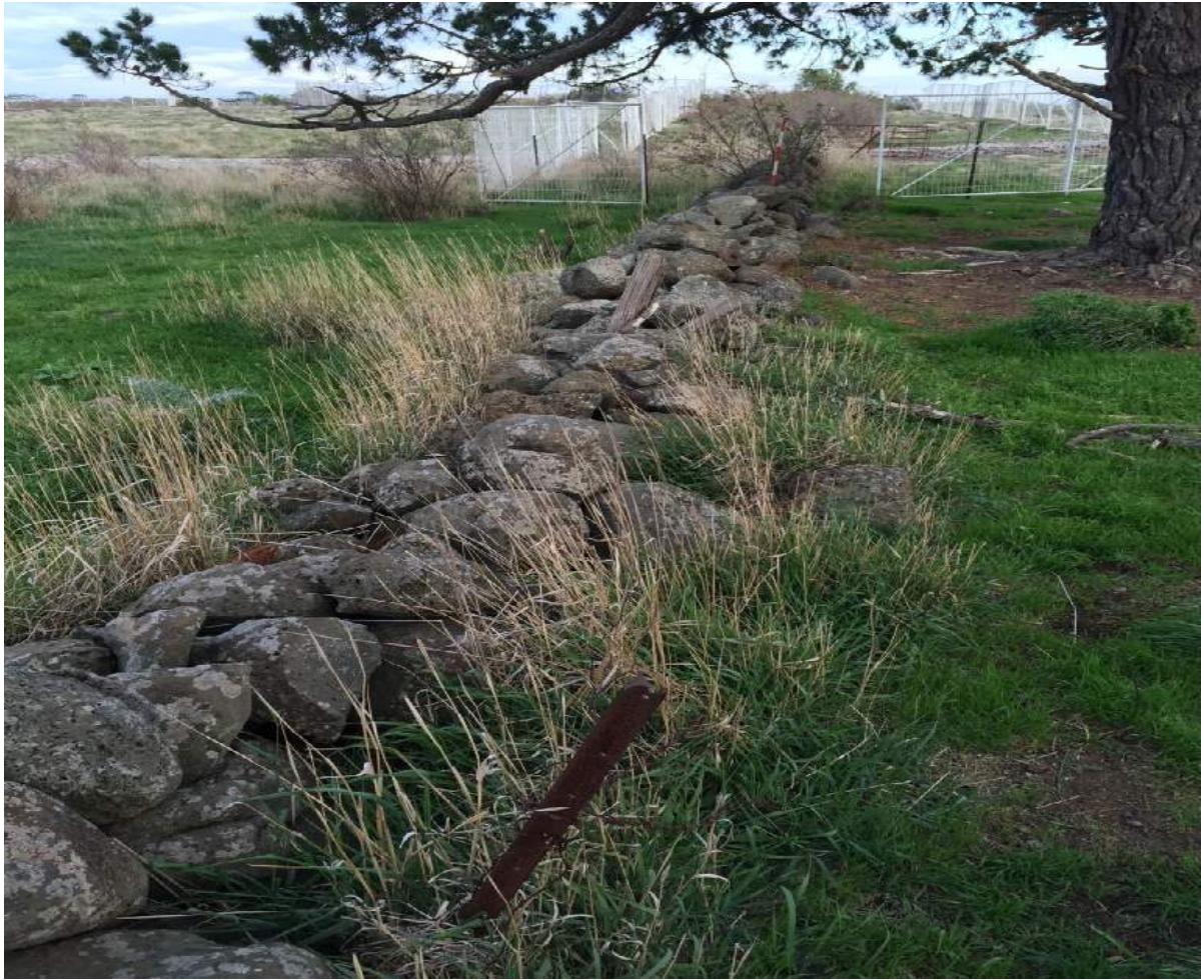
The eastern sections of Wall No 3 at 40 Dwyer Street Kalkallo looking west. This is a low composite wall and a remnant timber is visible mid frame (27/5/15 Photo R.J. Marshall)
