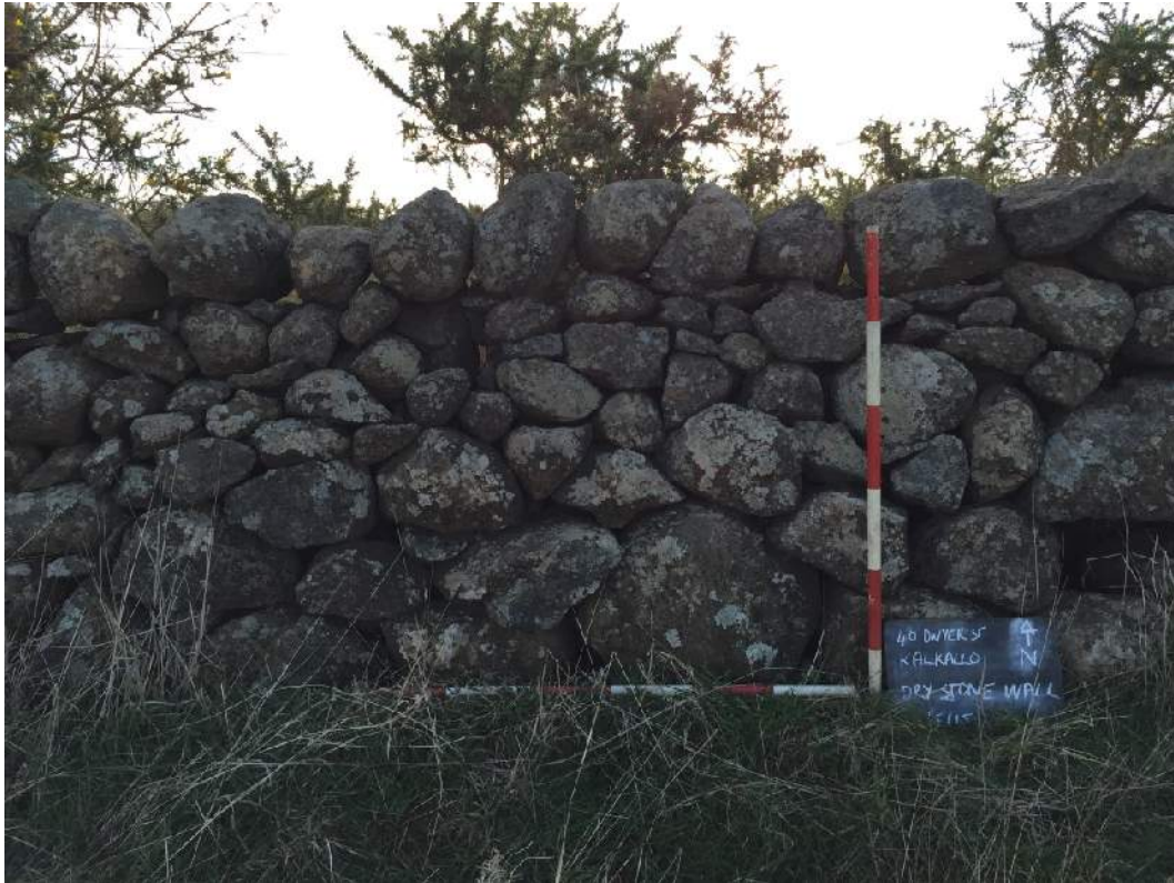
Section 1 of the east-west dry stone wall at 40 Dwyer Street Kalkallo showing detail of the coursing. Note the larger size coping stones over courses of smaller stone (27/5/15 Photo R.J. Marshall).
