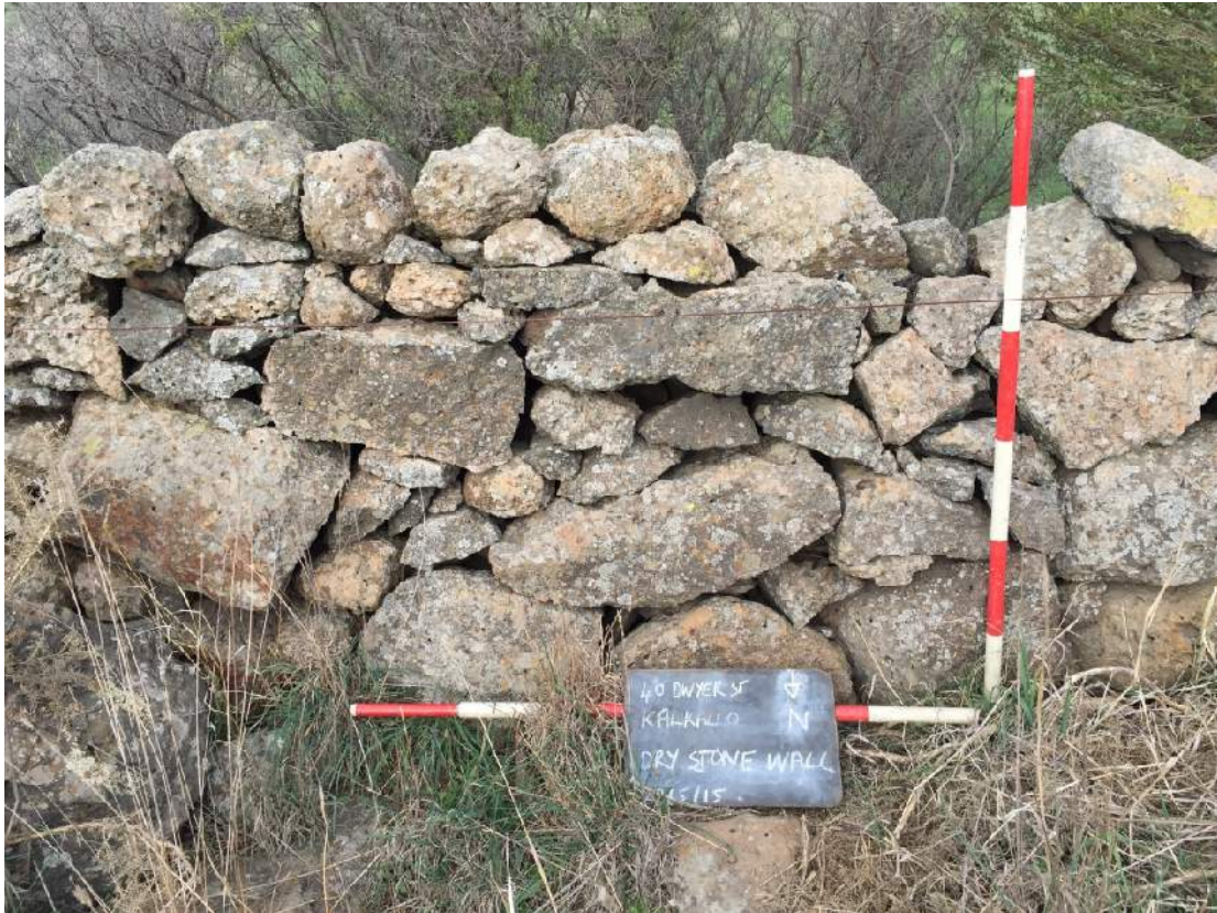
Section 1 of the east-west dry stone wall at 40 Dwyer Street Kalkallo showing detail of stones (middle frame) that have been altered, possibly faced (27/5/15 Photo R.J. Marshall).
