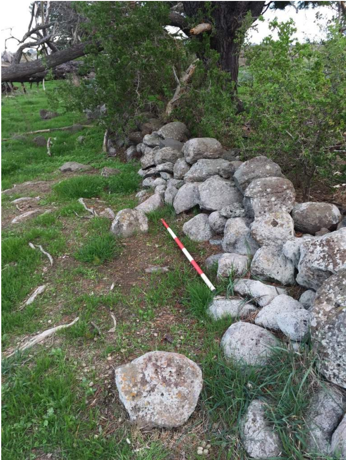
Plate 4. A section of Wall 3 of the east-west dry stone wall at 40 Dwyer Street Kalkallo. This is a poorly preserved part of the wall close to the Merri Creek floodplain and is a combination of aligned and tumbled rocks (27/5/15 Photo R.J. Marshall).
