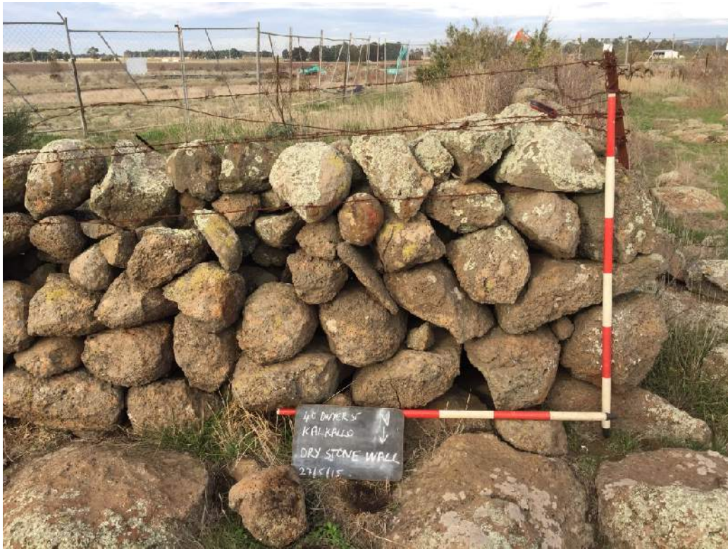
Wall 3 at 40 Dwyer Street Kalkallo its western end where it heads south to join wall No 2. Note the rough construction and the addition of the wire and star pickets (27/5/15 Photo R.J. Marshall).
