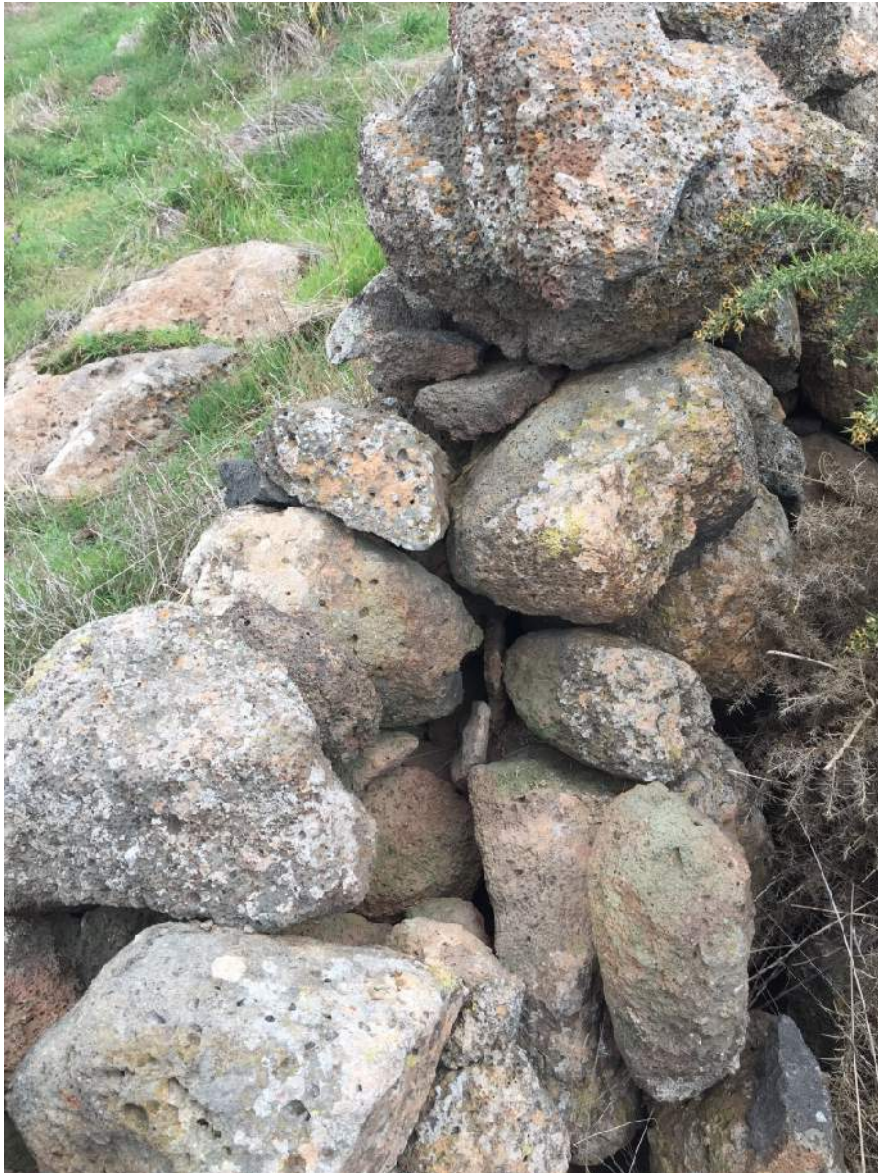
Collapse section of Section 1 of the east-west dry stone wall at 40 Dwyer Street Kalkallo showing infilling (27/5/15 Photo R.J. Marshall).
