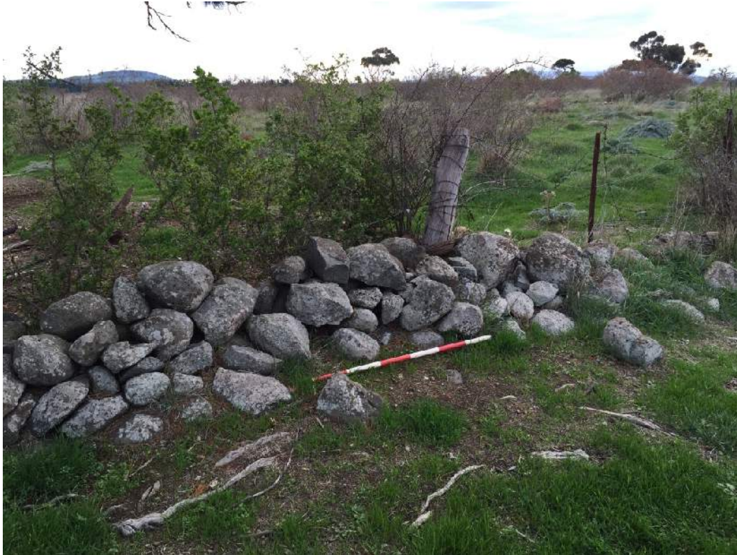
Wall 3 of the east-west dry stone wall at 40 Dwyer Street Kalkallo. This is a collapse section of a former composite wall. Note the corner timber post and recent wire and star picket additions. (27/5/15 Photo R.J. Marshall).
