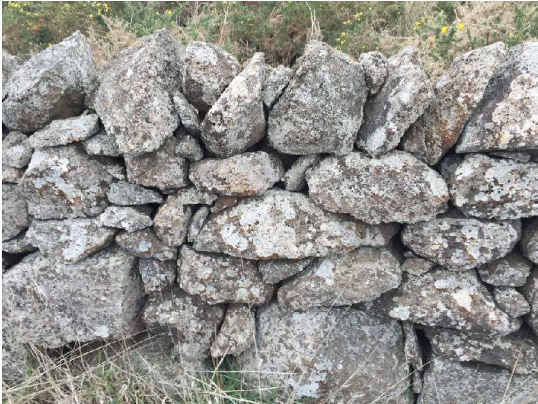
Section 1 of the east-west dry stone wall at 40 Dwyer Street Kalkallo. This is a detail showing the coping stones and plugging (27/5/15 Photo R.J. Marshall).
