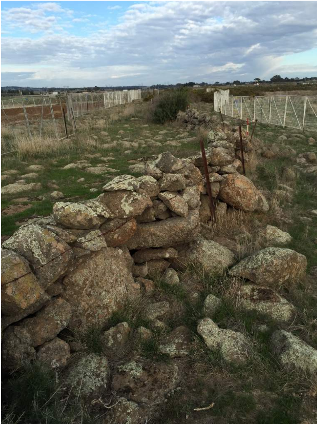
Plate 3. Wall 2 of the east-west dry stone wall at 40 Dwyer Street Kalkallo. This photo is looking in a southwesterly direction along the wall which has been protected from the nearby construction with some temporary fencing. Note the tumble of rocks in the foreground and the star picket and barb wire fence along its northern side indicating that whilst still a rural property the wall was no longer stockproof (27/5/15 Photo R.J. Marshall).
