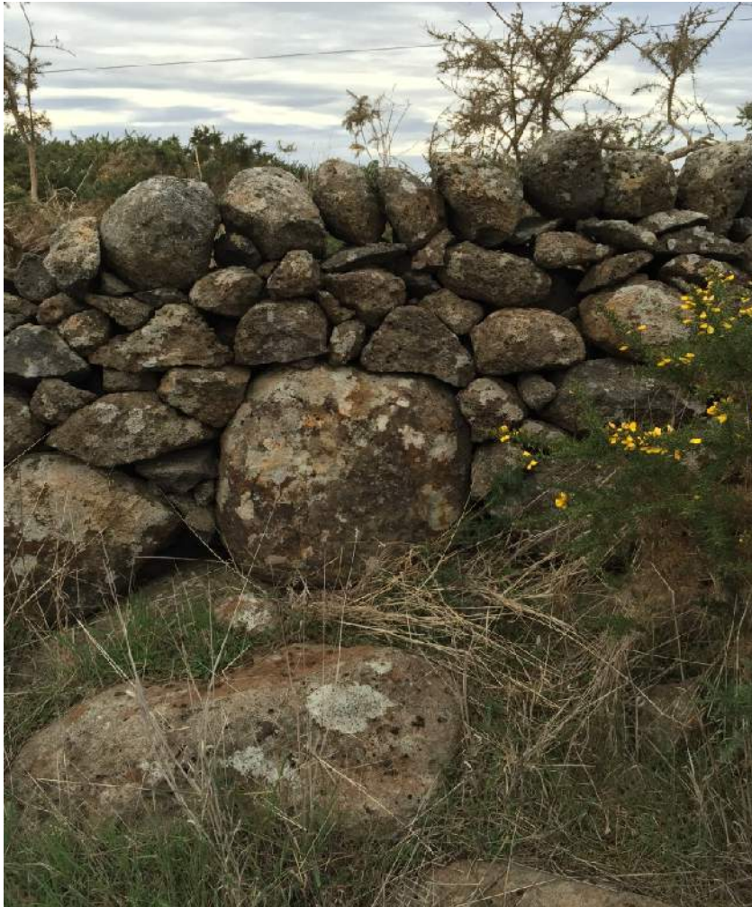
Section 1 of the east-west dry stone wall at 40 Dwyer Street Kalkallo showing the contact between the foundation stones and the underlying stony rise (27/5/15 Photo R.J. Marshall).
