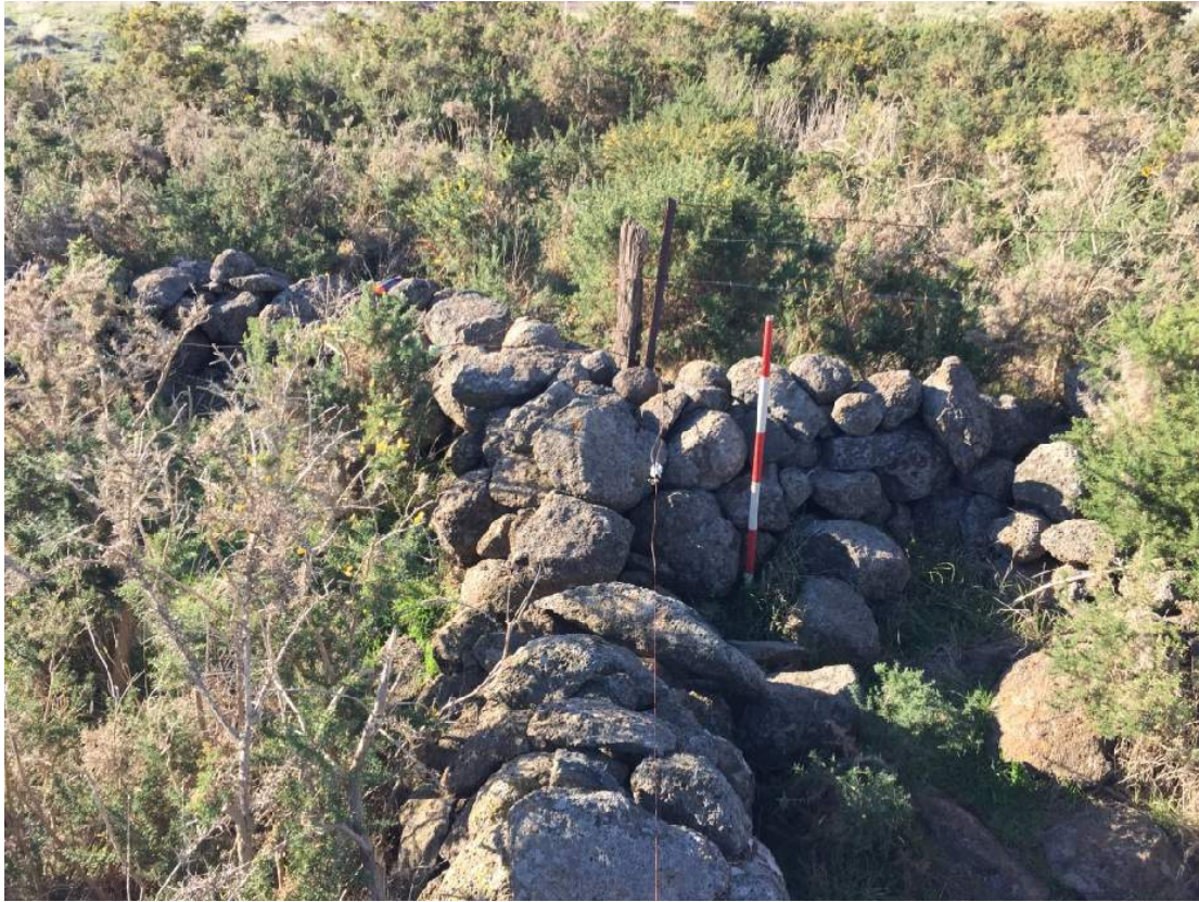
Plate 2. Intersection of wall Sections 1 and 2 of the east-west dry stone wall at 40 Dwyer Street Kalkallo. At this intersection the east-west wall heads north. The wall on the RHS of the frame is the northern end of a north-south dry stone wall which is a composite wall. A remnant timber post is visible in the middle frame (27/5/15 Photo R.J. Marshall).
