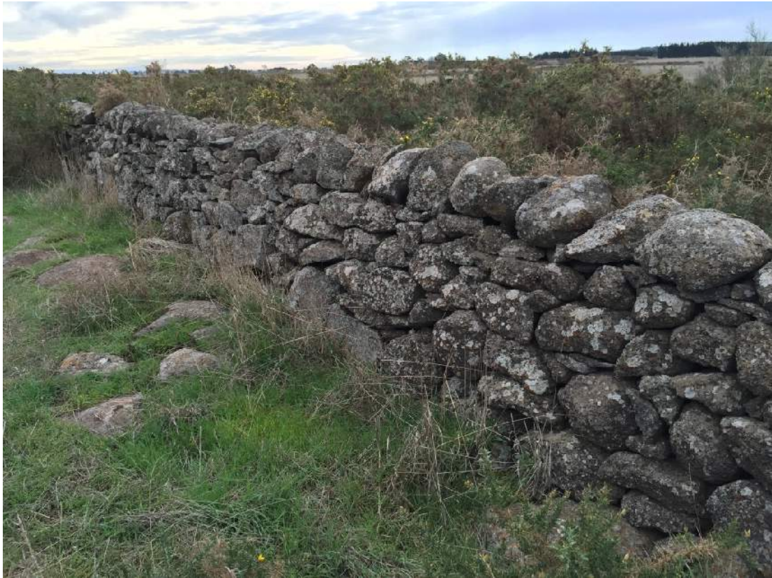
Plate 1. Section 1 of the east-west dry stone wall at 40 Dwyer Street Kalkallo. This is a well preserved part of the wall as the coping and plugging stones are in place. The stony rise is visible as rocks in situ in the ground (27/5/15 Photo R.J. Marshall).
