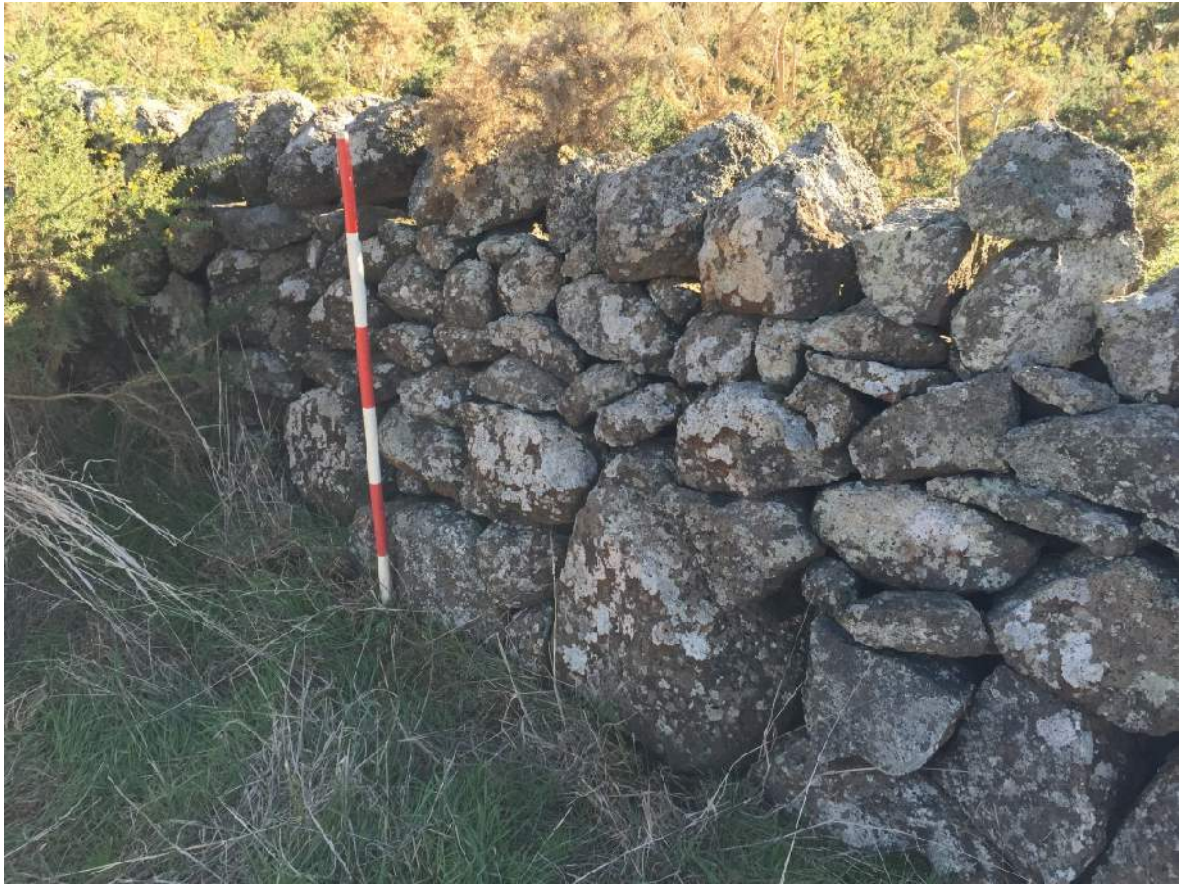
Section 1 of the east-west dry stone wall at 40 Dwyer Street Kalkallo showing detail of the coursing on the southern side (27/5/15 Photo R.J. Marshall).
