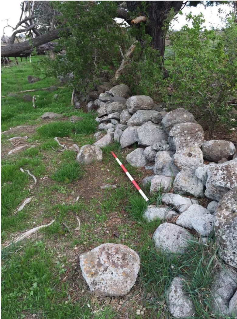
Partially collapsed section of Wall No 3 at 40 Dwyer Street Kalkallo near its eastern end looking along the alignment (27/5/15 Photo R.J. Marshall).
